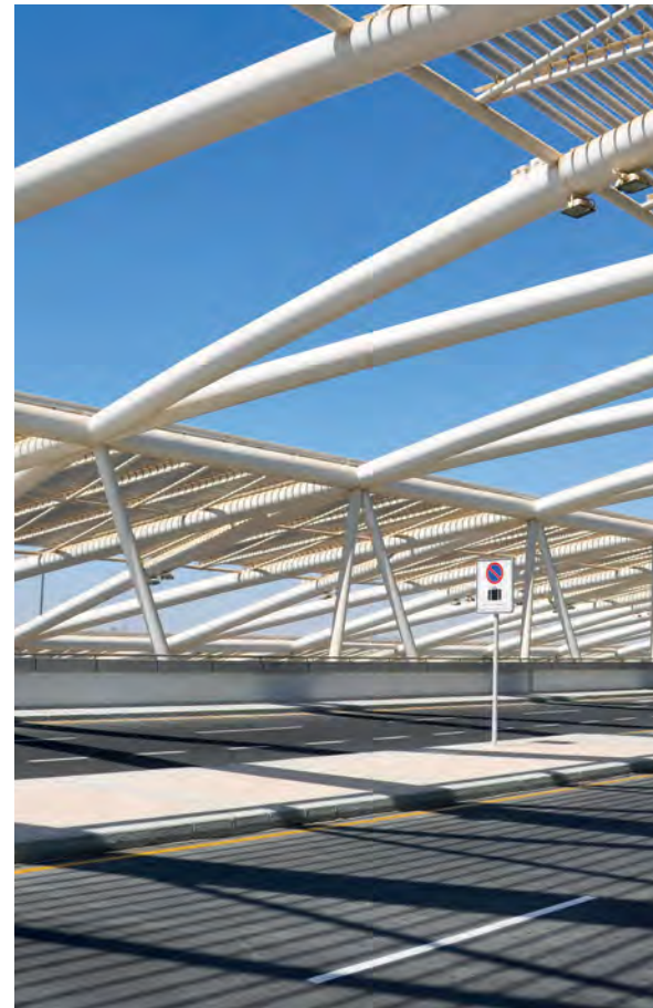
Cairo International Airport, Terminal 3 – protected by SteelMaster
